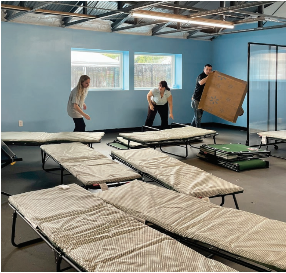
Left: Skidmore students played an important role alongside RISE staff and volunteers in preparing the new 24/7, low-barrier homeless shelter on Adelphi Street in Saratoga Springs, helping to assemble beds, paint walls, and create welcoming, functional spaces for guests.
